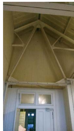
Former 3rd floor Room Divisions
